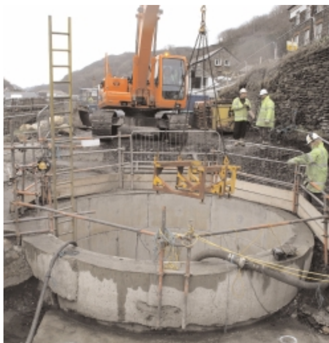
Tunnelling equipment is lowered into the south shaft
